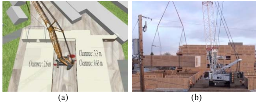
Figure 13. Crane Clearances: (a) from Visualization Model, (b) from Construction Site
