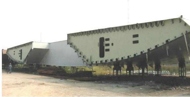
Figure 3: Typical steel deck segment of the bridge
