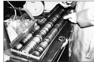
device for clamping nozzle parts
